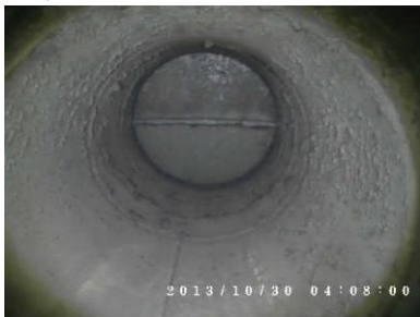
Still image taken from front camera in a 300mm diameter round duct.
